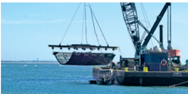
Muro marino de Hereford Inlet - North Wildwood, NJ
