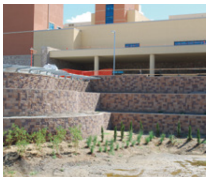
Hospital St. Anthony – Denver, Colorado
